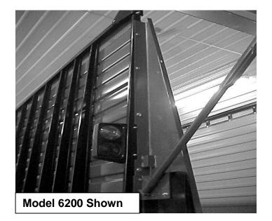
Drill 13/32" diameter hole on inside bottom corner and bolt tight using 3/8 x 2" machine bolt and 3/8" spin locknut. Do not over tighten. (See photo below.)
