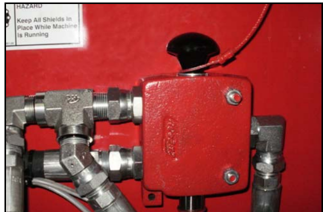
Figure 4. Emergency Trip Cable - Hydraulic Selector Valve
